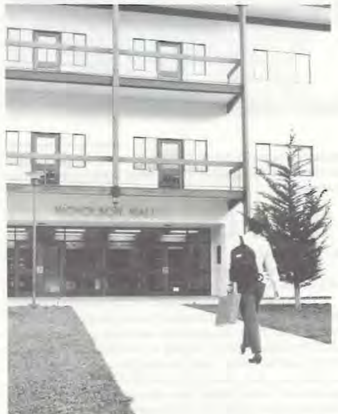
Photo by PH2 Ken Trent Nicholson Hall, one of DLI's newest general instructional facilities, provides students a comfortable academic environment and some of the most up-to-date equipment available.
