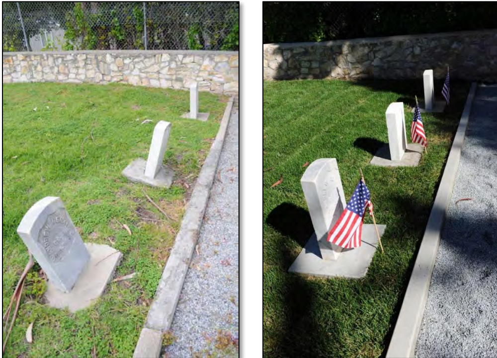
Figure 49 – Before and after photos of the $313,000 cemetery project, 2010. Left Photo by Al Macks. Right Photo by Hiro Chang.
