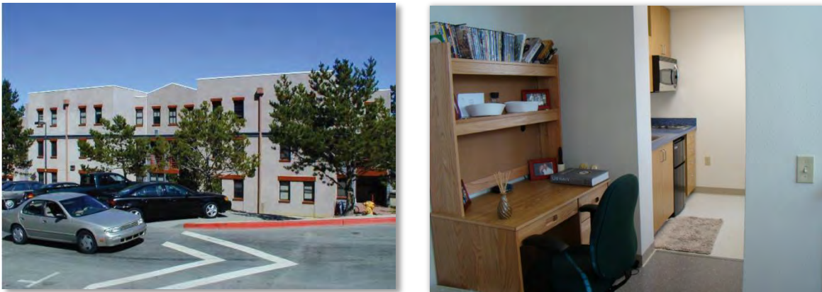
Figure 48 – Kitchens were added to Presidio of Monterey barracks rooms, including sinks with garbage disposals, microwave ovens, and two-burner electric ranges, 2008-2010.
