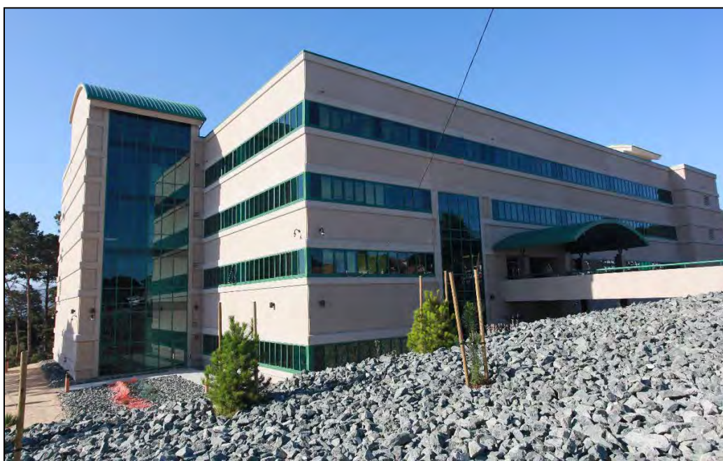
Figure 12 – Building 417, Khalil Hall, despite landscape challenges, became operational in 2010.
