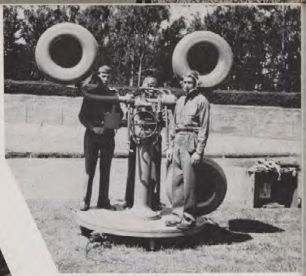
The Army Day display includes Coast Artillery equipment. This is a sound locator for spotting the distance and direction of approaching planes.
