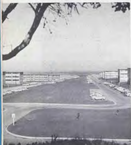
New barracks completed
