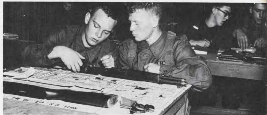
The trigger housing group
