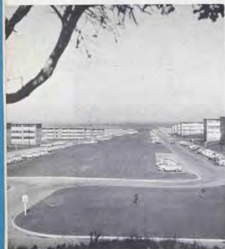
New barracks completed
