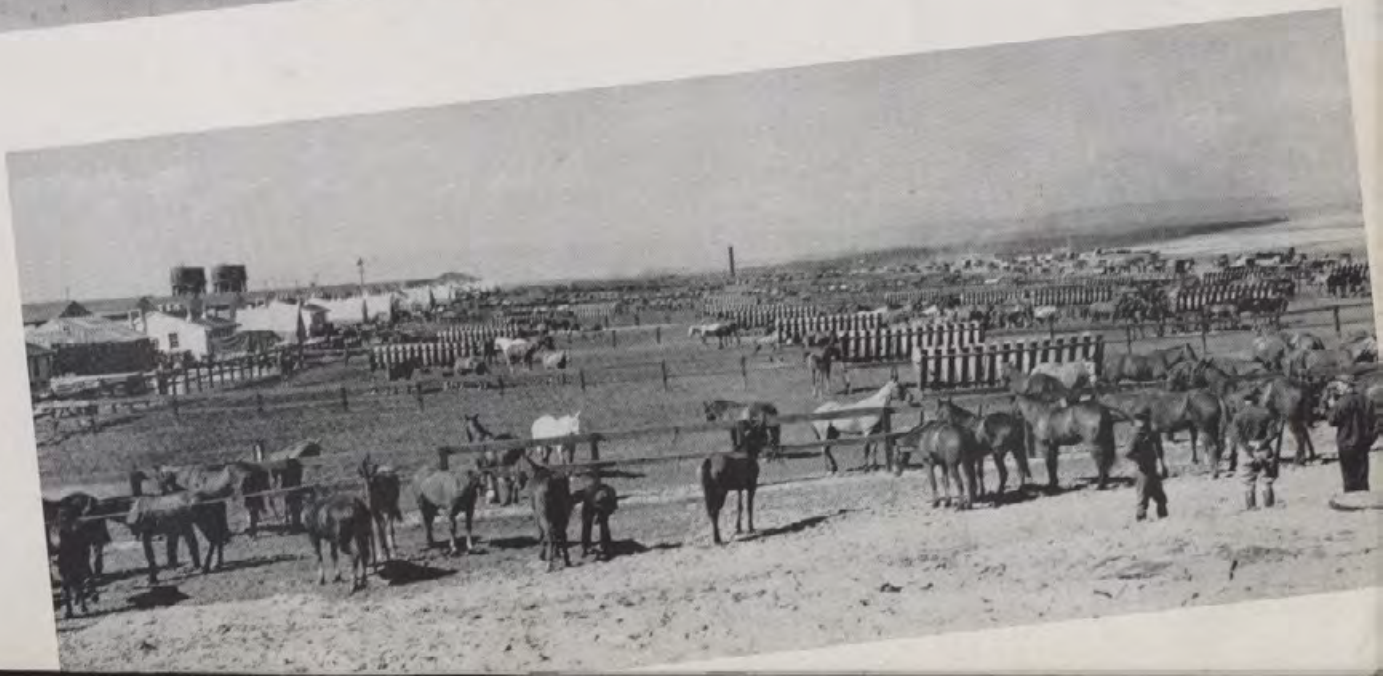
The view at right shows Field Artillery corrals, set away from the main part of the Division area.
