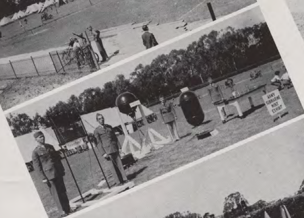
The Army Day display includes Coast Artillery equipment. This is a sound locator for spotting the distance and direction of approaching planes.
