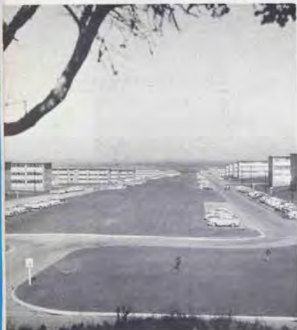
New barracks completed
